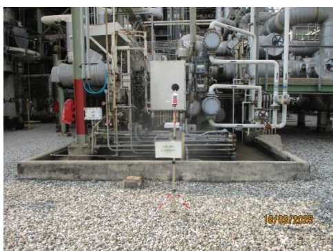
Hydrogen Compressor (R-401)
